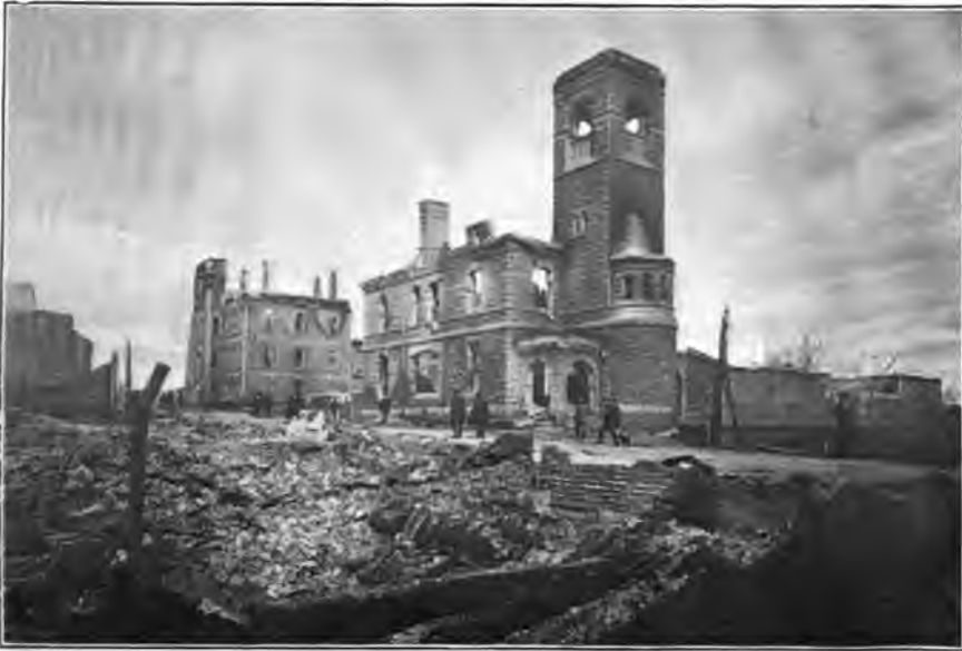
PHOTO. BY PITTAWAY. THE HULL POST OFFICE AND COURT HOUSE.
